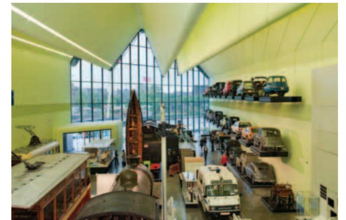
The Riverside Museum has triple-thickness glass that helps stabilise the environment within the building and conserve heat. The glazing is heavy-filtered and contains solar-gain which helps the building's heating and cooling systems maintain a stable environment © Culture and Sport Glasgow (Museums)
