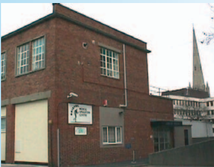
Figure 2 Outside the first BMSC building
