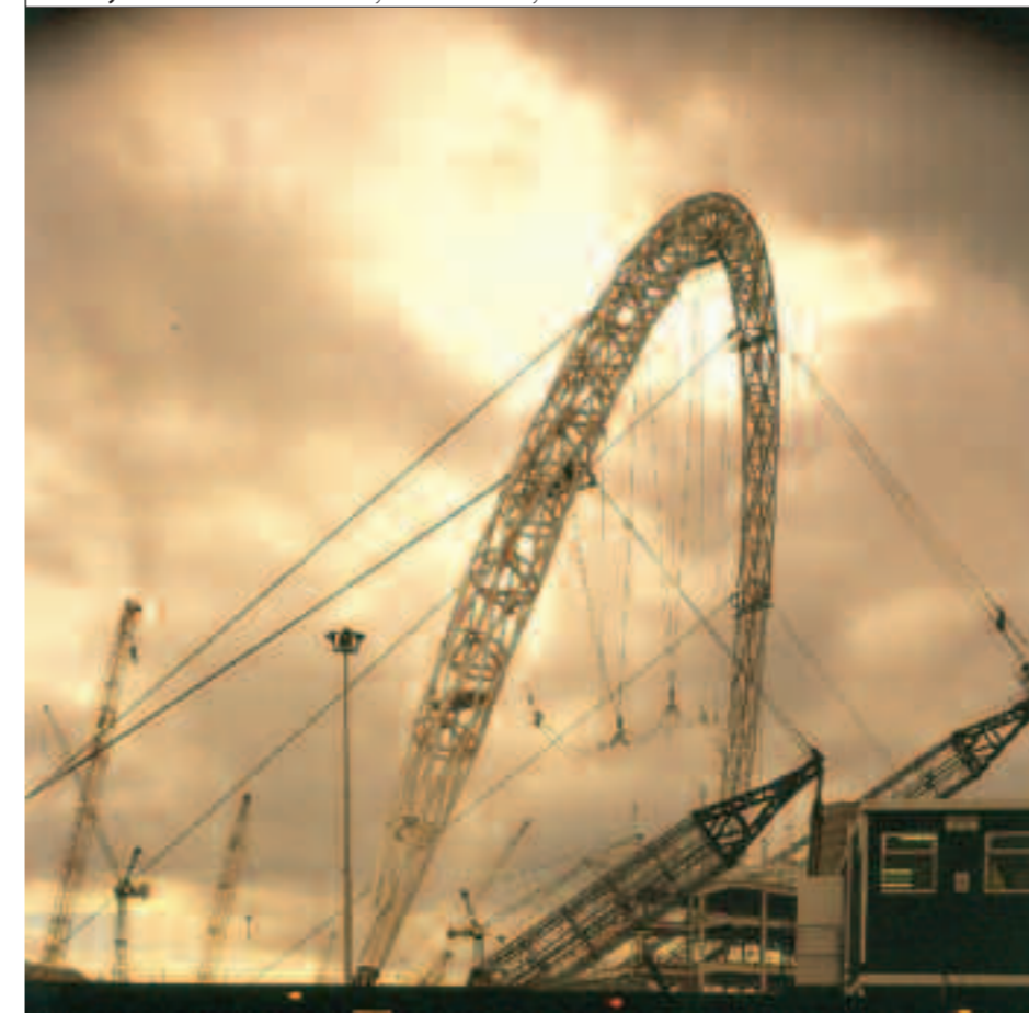
Wembley Stadium main arch Courtesy of Bianchi Morley
