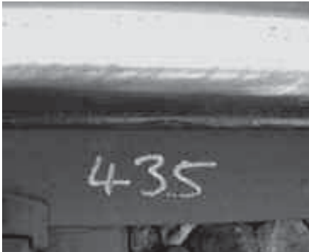
An example of gauge corner cracking on a 900m curve high rail
