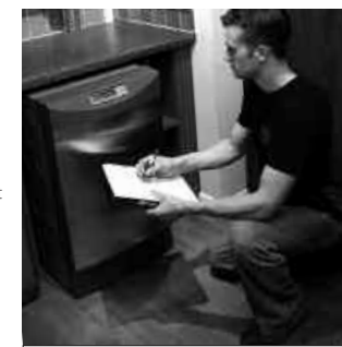
A micro-CHP unit, replacing a floor-standing central heating boiler © Powergen
