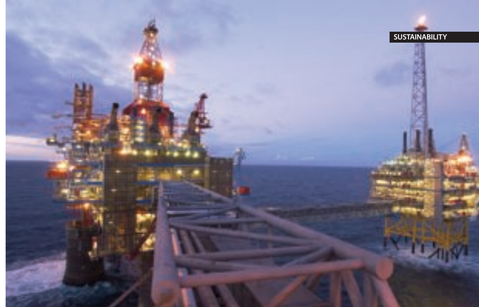
Statoil's Sleipner CO 2 disposal installations in the North Sea © Bitmap
