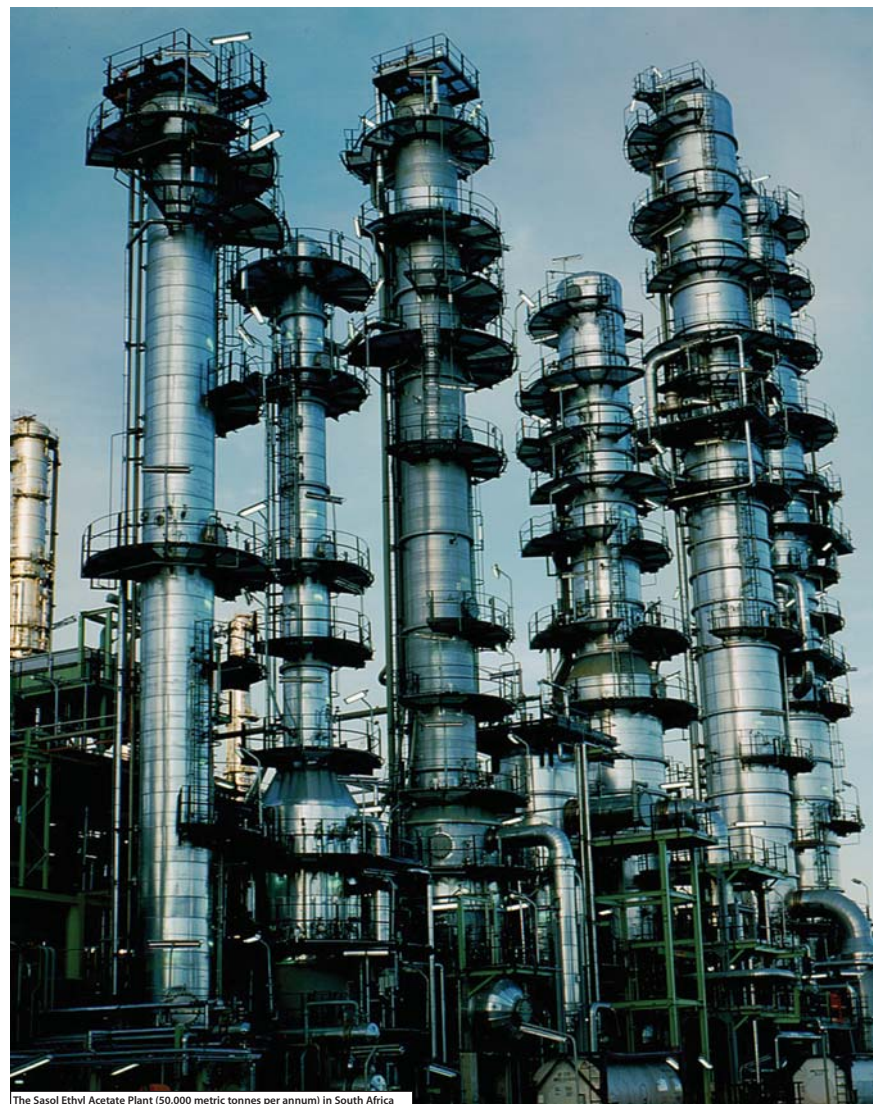
The Sasol Ethyl Acetate Plant (50,000 metric tonnes per annum) in South Africa
