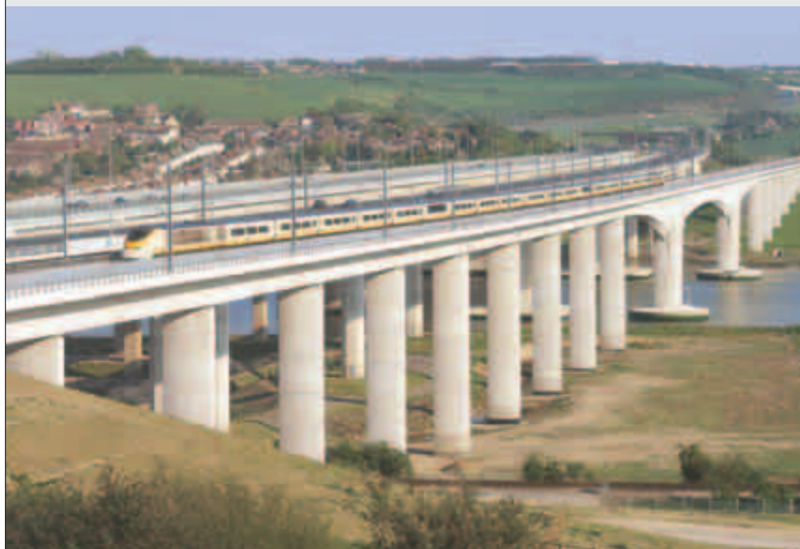
Medway Bridge © Central Photography
