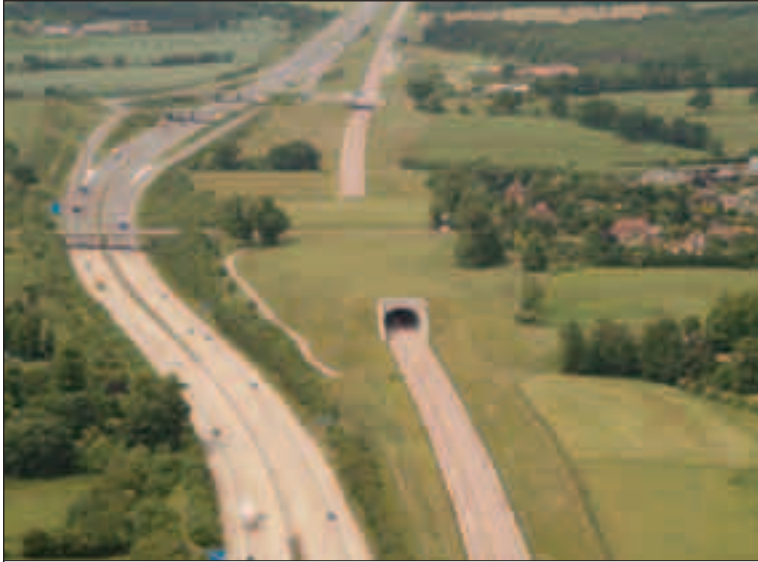
Eyhorne Street cut and cover tunnel © Mac Hawkins/LCR
