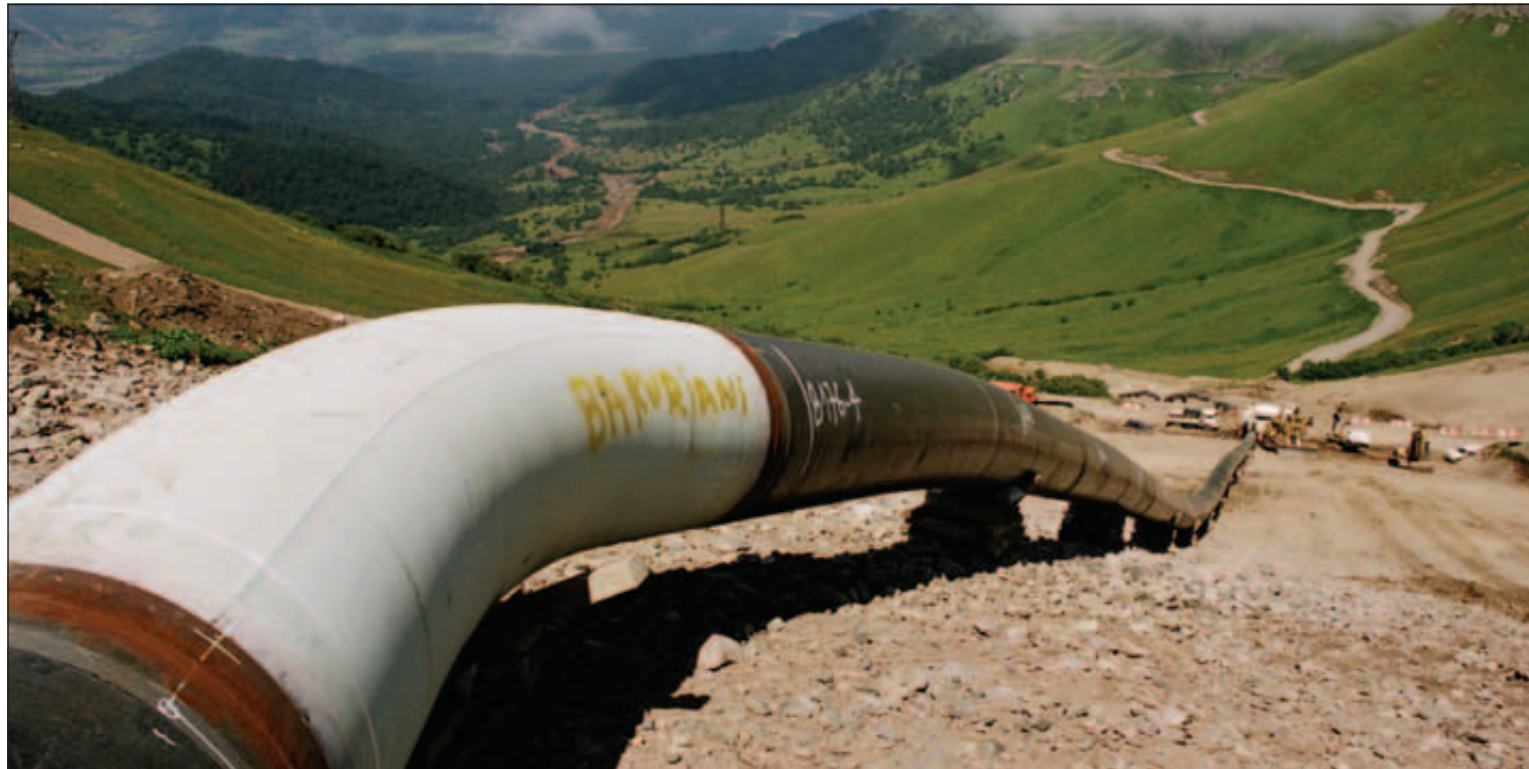
Pipeline construction on severe gradients, Georgia, August 2004 © BP plc
