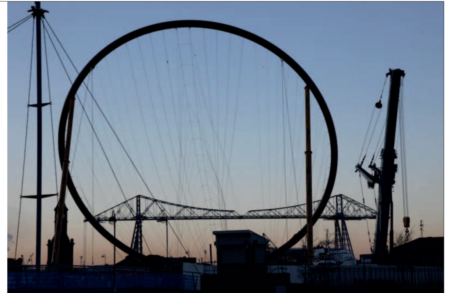
The Temenos rings were raised into place in February 2010. The Middlesbrough Transporter Bridge can be seen in the background © Kirstie Handley Photography/Teess Valley Regeneration
