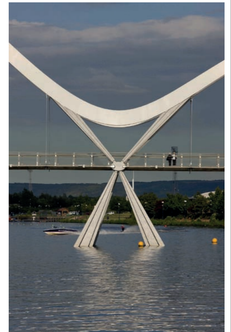
The central support. Compression forces are taken from each of the arches through the arms to tie cables connected to the central one © Morley von Sternberg
