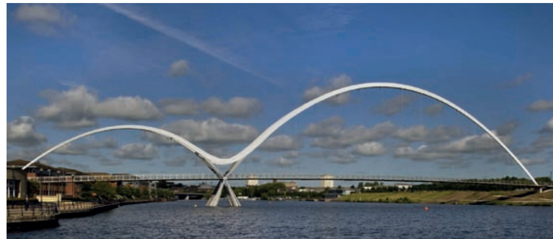
The Infinity Bridge, Stockton-on-Tees. The arches of the Infinity Bridge form a double span across the river. A reflex piece between the two arches holds them together making the two arches one continuous curve. The arch form, reflected in the still Tees, provides the origins of the bridge's name
