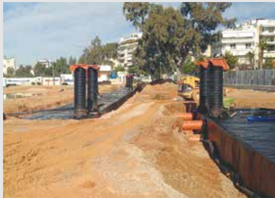
Onsite surface water attenuation is provided throughout the park in the form of geocellular tanks and deep gravel trenches. Both act to store water during times of heavy rainfall, which protects the municipal drainage system from being overloaded and allows for infiltration to recharge the aquifer © Michel Denancé
