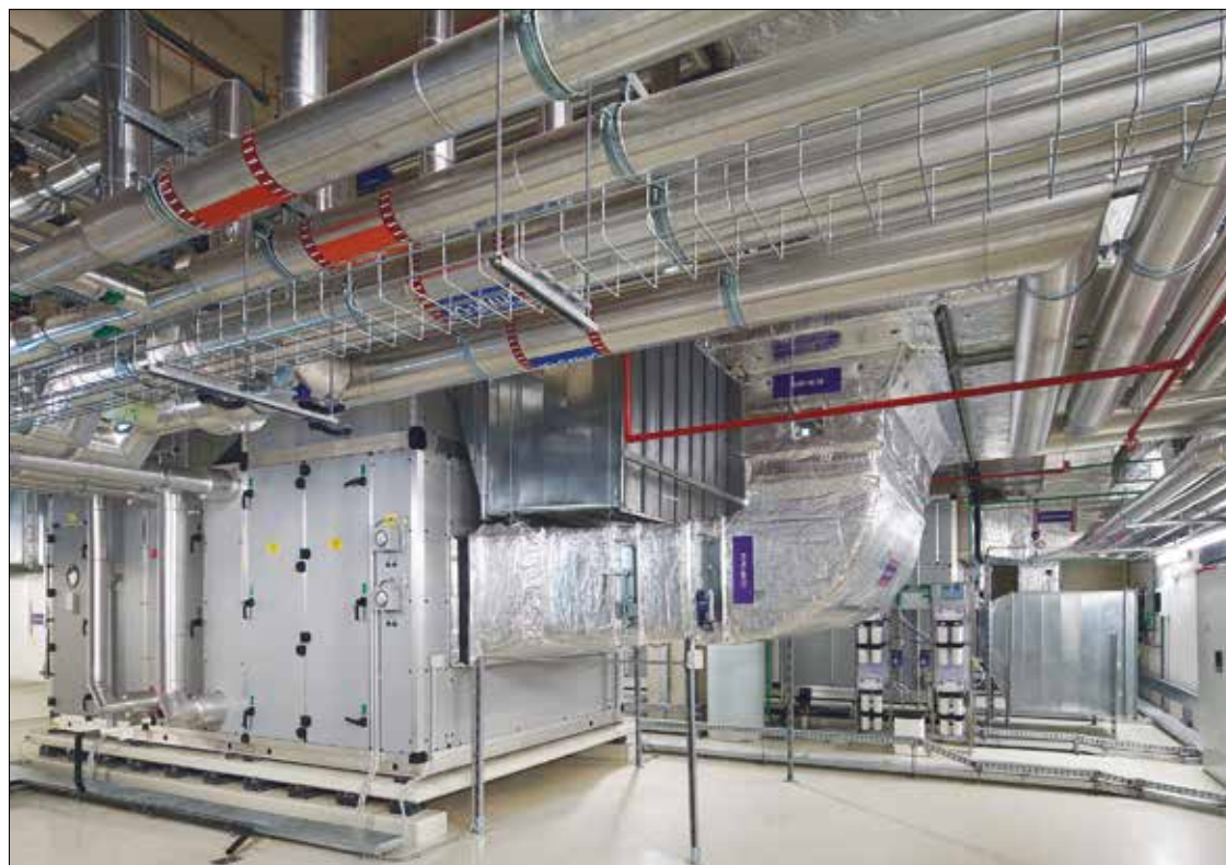
The air-handling unit supplying conditioned air into the opera theatre. The large ducts require lower air velocity and smaller fans, resulting in less noise close to the auditorium © Michel Denancé
