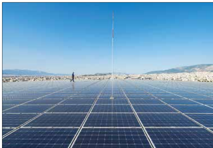
The tight packing of PV cells on top of the canopy was achieved by laminating the panels so that they can be walked on, which removes the need for maintenance walkways © Michel Denancé
