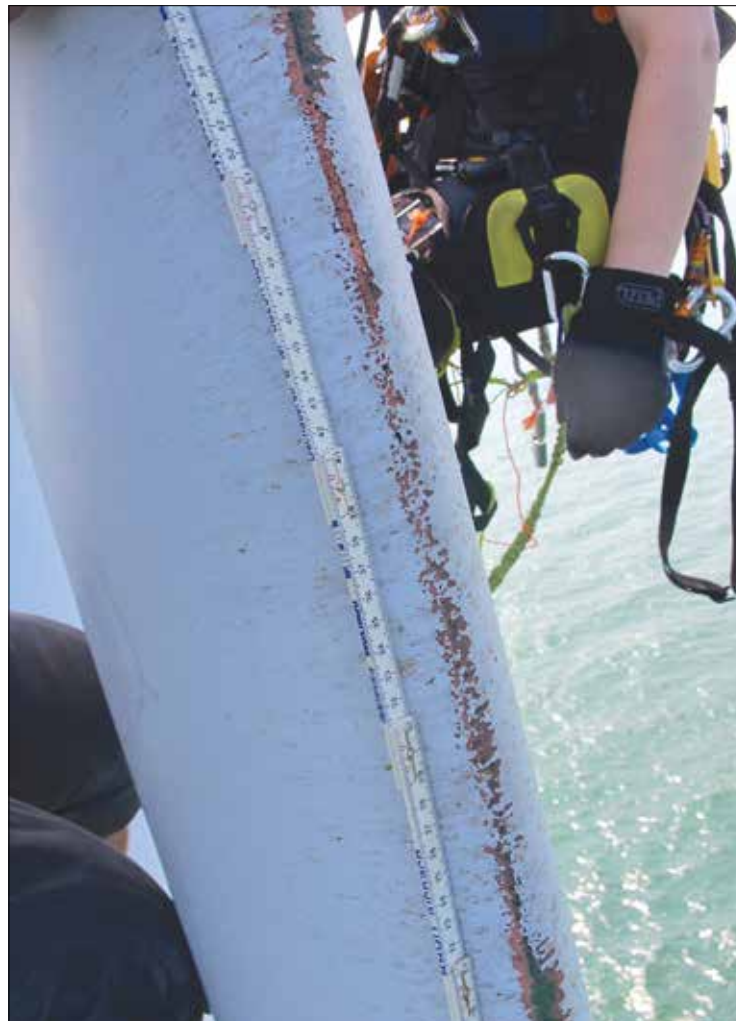
Blade leading-edge erosion is one of the key challenges facing the offshore wind industry. Leading-edge erosion is accelerated offshore because of harsher environmental conditions and can prove costly for offshore wind farm owners and operators, through lost power generation and revenue
