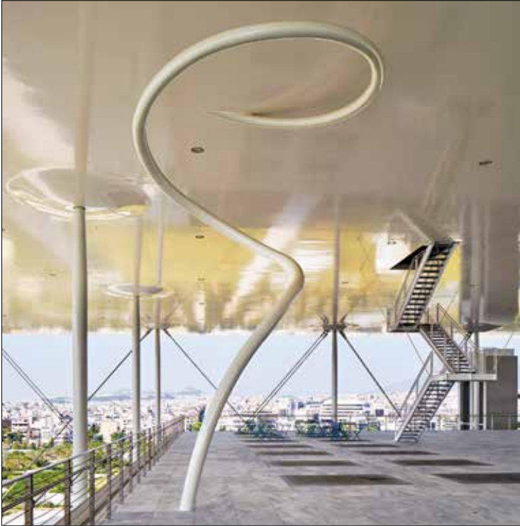
A particular challenge was how to run a large and inflexible high-voltage cable down from the PV cells on the canopy, invisibly and allowing for the large movements of the roof. The solution was an elegant spiral sculpture, which happens to support and contain the cable and effectively absorbs any movement © Michel Denancé
