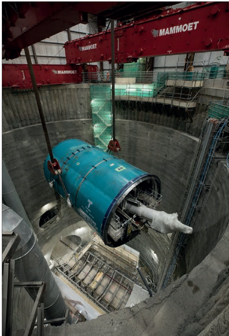
The front end of 'Rachel', the tunnel boring machine (TBM) driving the western section of the main tunnel, being lowered down the shaft at Fulham. Tideway's six TBMs are each named after an inspirational woman from the local area, chosen by the public from a shortlist. The name 'Rachel' commemorates the pioneering engineer Rachel Parsons, daughter of Sir Charles Parsons, the inventor of the steam turbine. During the First World War she replaced her brother as a director of her father's company. She was founder President of the Women's Engineering Society ( Ingenia June 2019) and in 1920 co-founded the engineering company Atalanta Ltd in Fulham Road, where all the employees were women
