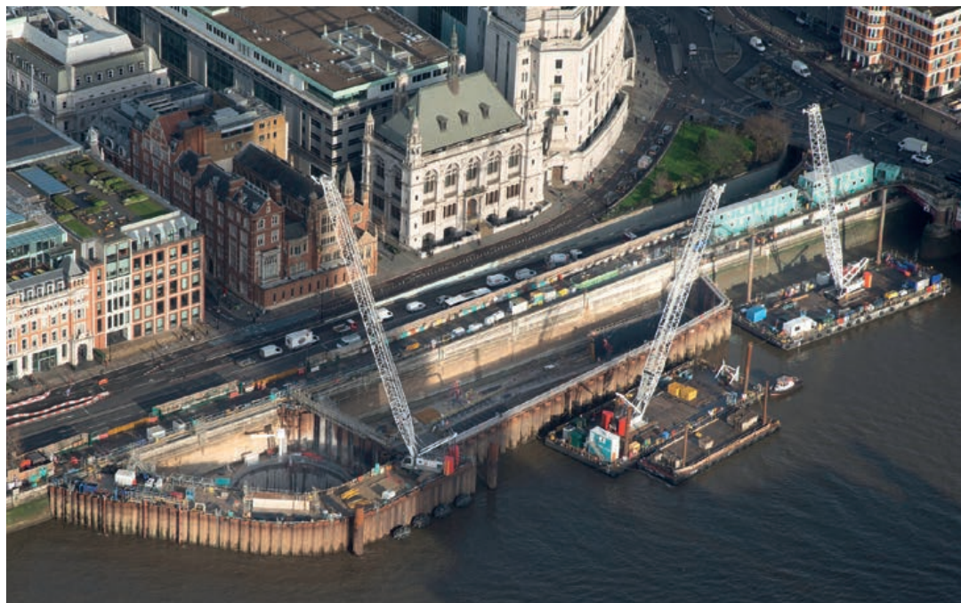
Blackfriars north foreshore. A 100-metre, 3,500-tonne interconnecting culvert will be the largest structure to pass along the Thames later this year. It will be lifted into the central section above and then connected to the CSO drop shaft – below the crane on the left of the picture © Tideway
