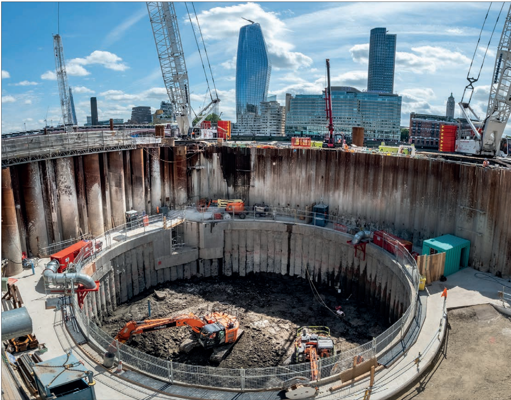
A cofferdam was constructed on Blackfriars north foreshore so that a dry workspace could exist below the level of the River Thames. A drop shaft has been designed to intercept both the LL1 sewer located within the listed Bazalgette river wall and the existing Fleet sewer outfall, which is located under Arch 1 of the Blackfriars Bridge, to the new Tideway tunnel. The shaft is now excavated to a depth of 23 metres and when completed will be 53 metres deep (to invert level) with an internal diameter of 22 metres © Tideway
