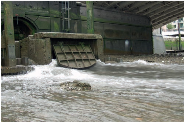
A combined sewer overflow releases rainwater and sewage during peak flows 60 times a year © Tideway
