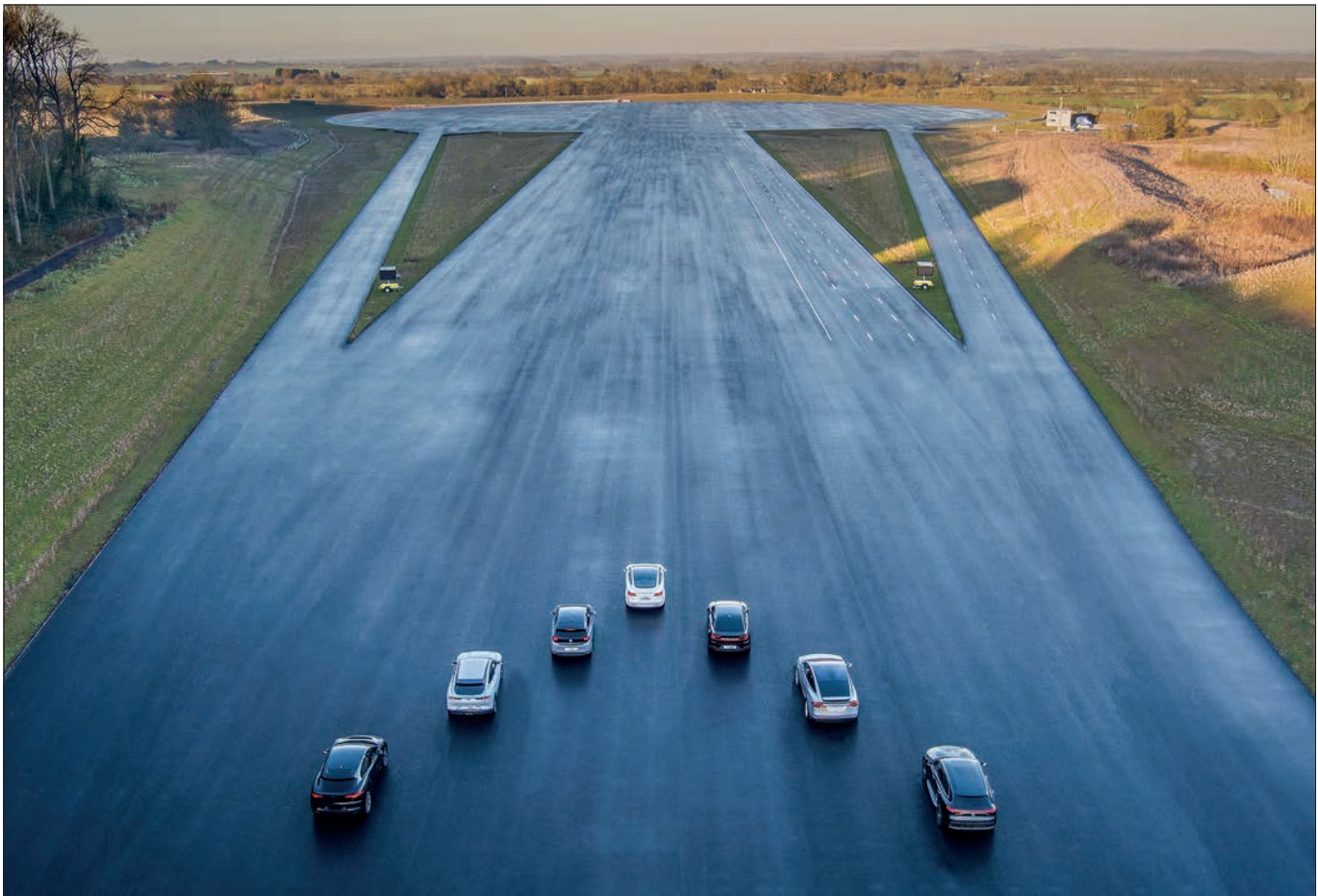
HORIBA MIRA's 'highway' facility has a fully configurable dynamic platform with an approach 15 lanes wide. It's used for testing a range of scenarios involving advanced driver assistance systems and connected and autonomous vehicles, such as lane merging, lane assist, platooning, and autonomous emergency braking © HORIBA MIRA
