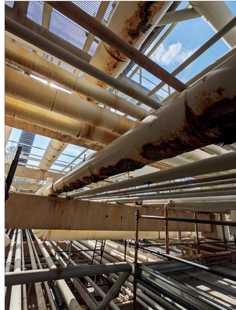
Pipe work at refineries is one of the places badly affected by corrosion under insulation. It can become visible at the bottom surface of pipes, where moisture is most likely to accumulate
