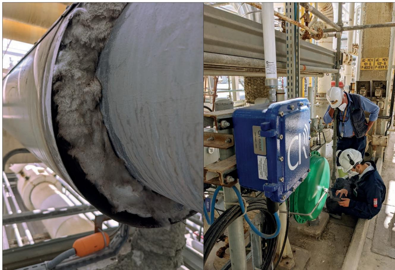
Left: Moisture sensors are fitted underneath insulation and metal cladding. Right: A control box that sends data from connected sensors to plant workers © CorrosionRADAR
