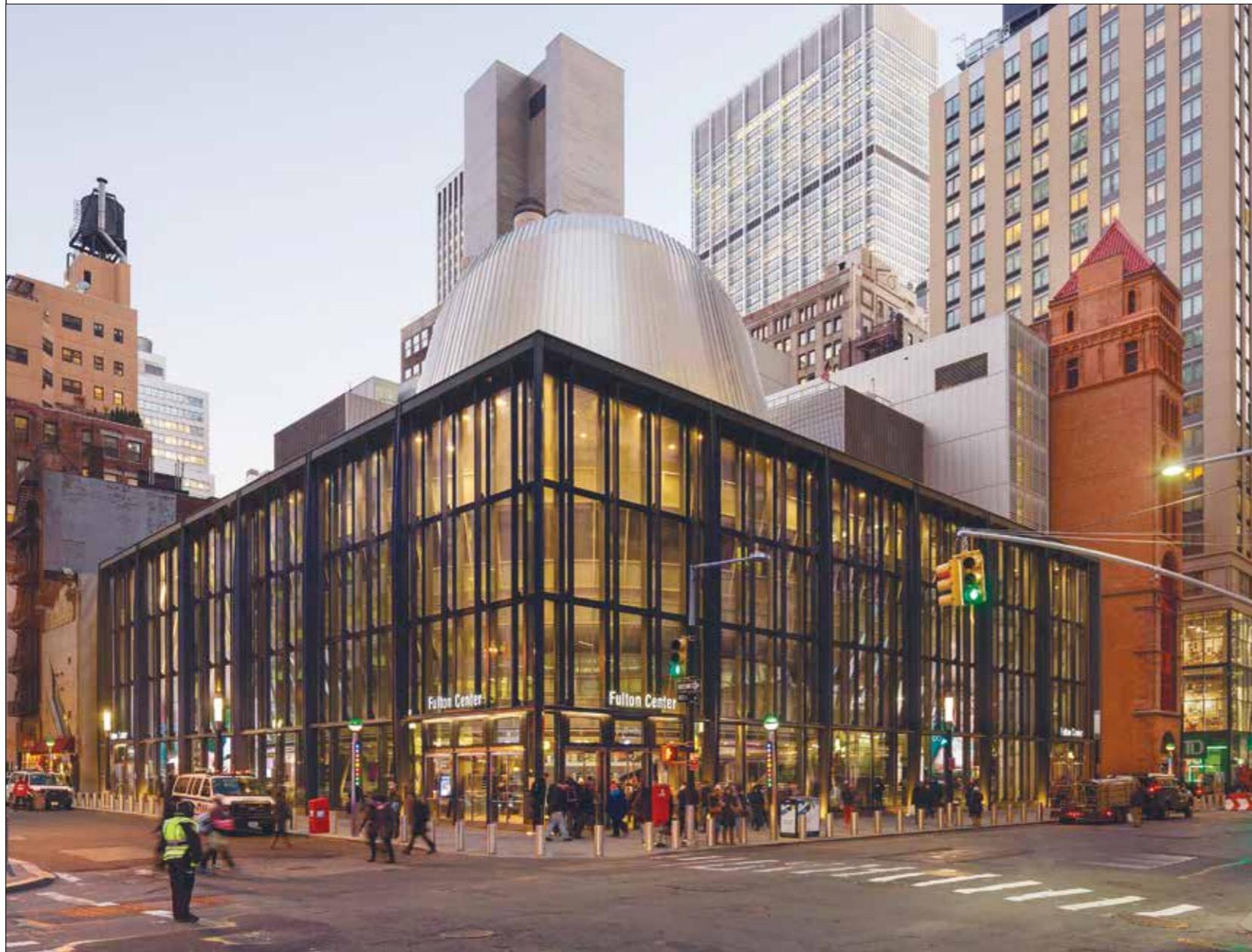
The northwest corner of the Fulton Center, showing the dome and the oculus rising above the steel and glass pavilion. At the rear is the west end of the Corbin Building projecting on to Broadway, with the eight-storey 'interstitial' building in between © James Ewing
