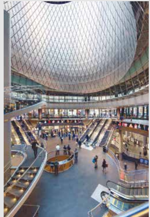
The new Fulton Center features open direct paths, widened corridors, and new mezzanines to separate entering, exiting, and transferring customers. The Sky Reflector-Net helps to draw light down from the inclined circular oculus deep into the subterranean levels of the Center, greatly reducing the costs of artificial lighting © James Ewing
