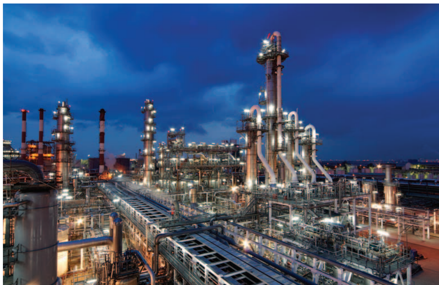
Alpha 1 plant, Jurong Island Singapore. This is the first-in-class plant using Lucite's Alpha technology. It was commissioned in the latter part of 2008 and cost $230 million to engineer and construct © Lucite International
