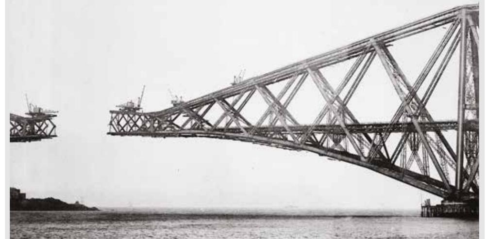
Construction of one of the beam sections that connect two of the Forth Bridge's giant balanced cantilevers in the 1880s © courtesy of the Institution of Civil Engineers
