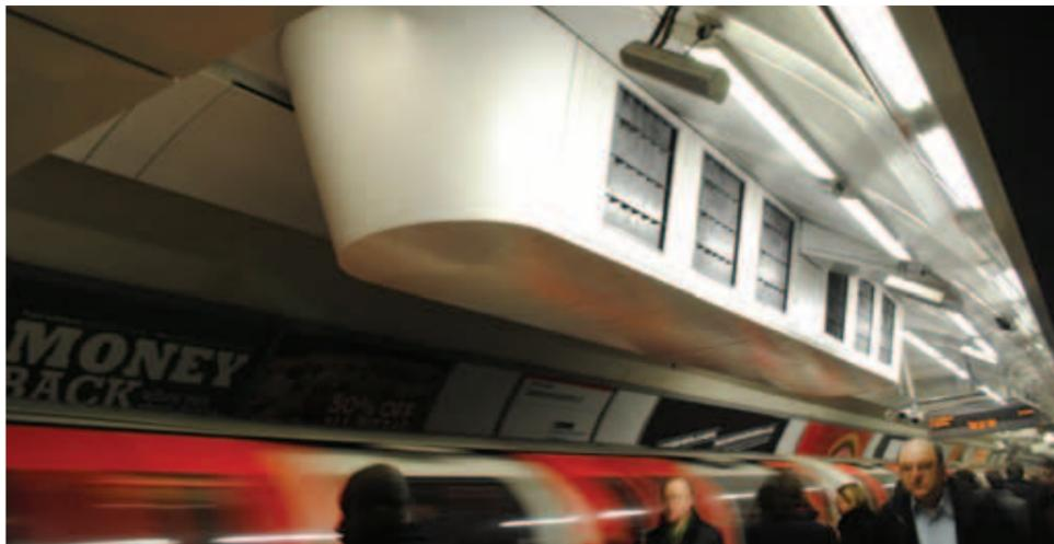
The air handling units *in situ* with coils, fans and other components supported by a frame, attached to a set of hangers suspended from lining rings on the tunnel roof
