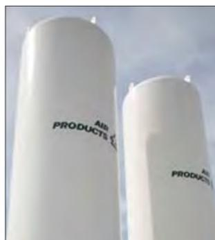
Using liquid nitrogen to cool makes the system intrinsically reliable. It means there is no compromise on sample storage temperature, -80°C is easily achievable. There is negligible power consumption and no waste heat. The system is almost silent in operation and no nitrogen is vented into the store; the waste gas is directed out of the building
