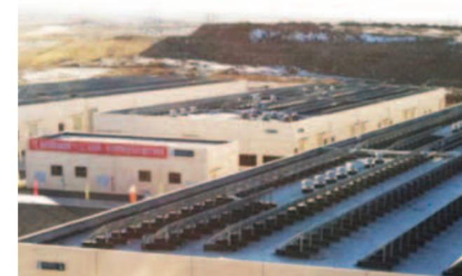
**BYD and the State Grid Corporation of China have built the largest grid battery storage facility in the world. Located in Zhangbei, Hebei Province, China, the LiFePO4 battery combines 140MW of renewable energy generation (both wind and solar), 36 MWh of energy storage and a smart power transmission system**
