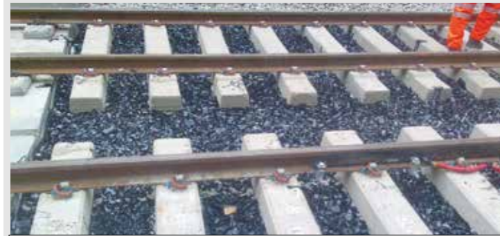
XiTRACK is used to solve a number of track quality issues to eliminate persistent and recurring maintenance problems. The ballast technology, using strong, tough, durable polyurethane, is the result of research carried out at Heriot-Watt and Edinburgh universities © Balfour Beatty
