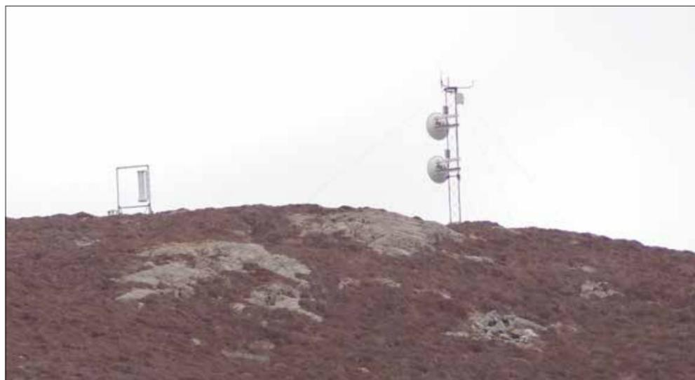
The wireless broadband link on the Shetland Islands uses antennas and masts to supply broadband rather than using phone lines. There is potential to extend the reach of the link in the future so there is the capacity for surrounding areas to access this fast connection © Shetland Broadband
