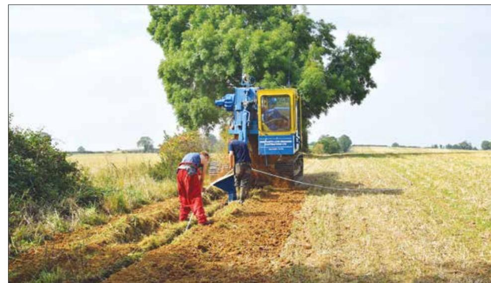
Volunteers in Abthorpe buried the fibre-optic cable between one and 1.5 metres below the earth to avoid disruption to the fibre if the 14-millimetre tube became waterlogged. They faced a challenging timeline because trenching work needed to lay the fibre had to be carried out in a two-week window between harvest and ploughing, so as not to disturb farmers © Tove Valley Broadband
