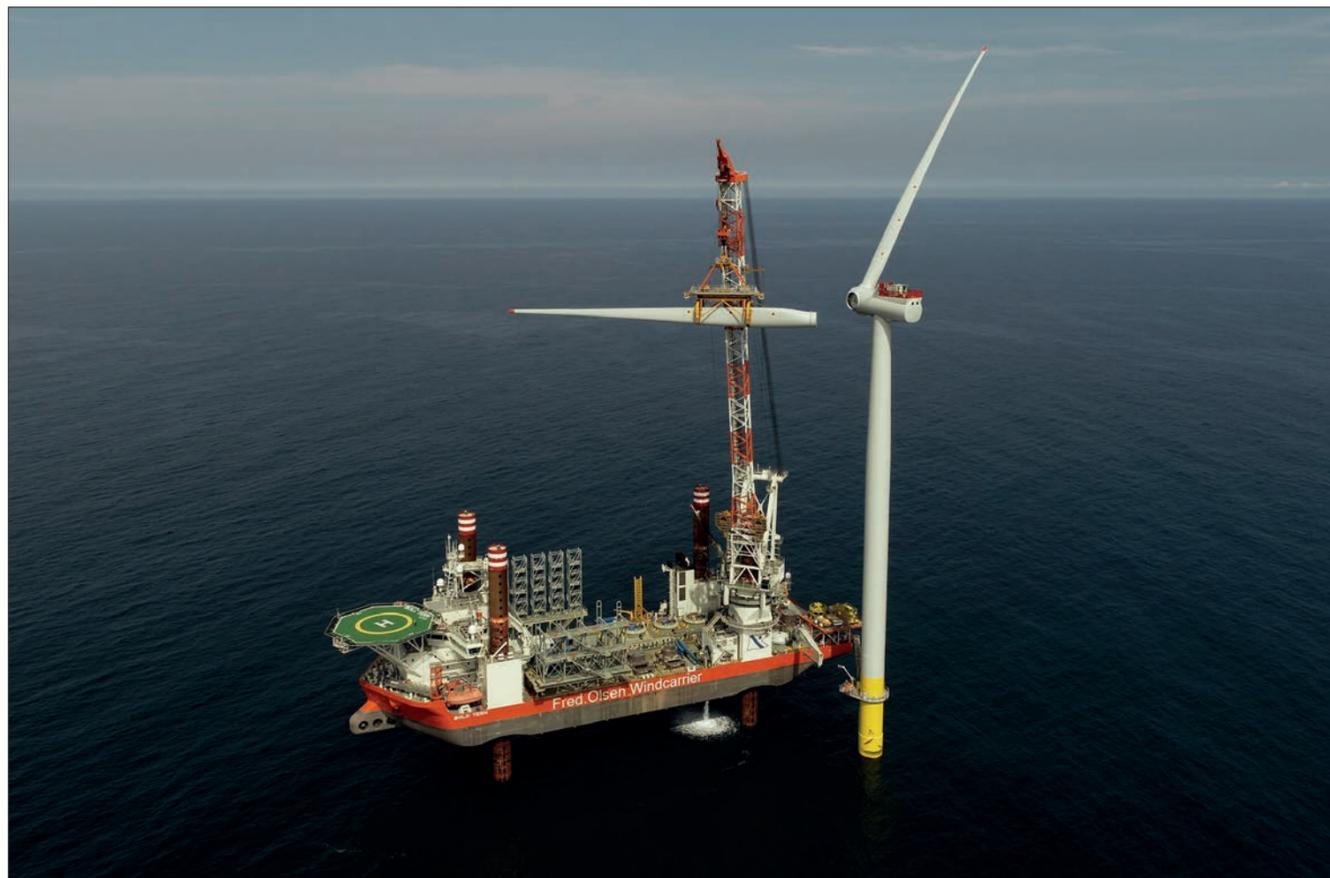
A jack-up barge that has sailed from Hull port with the components on board places its legs on the seabed to secure and lift the vessel so that it can install the blades and components © DEME group
