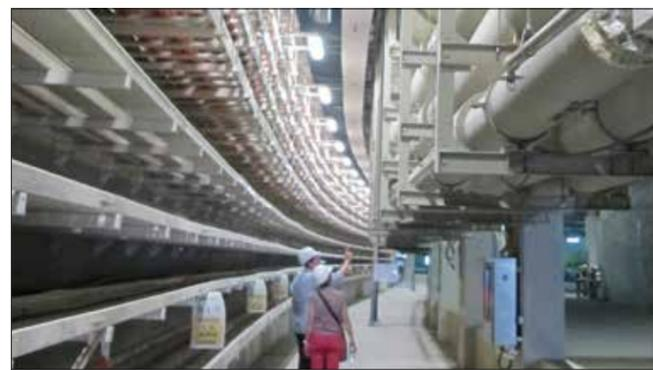
Cable trays and piping line the walls of the main service tunnel between the energy centre and the dome, part of the Gardens' large area of underground plant and services
