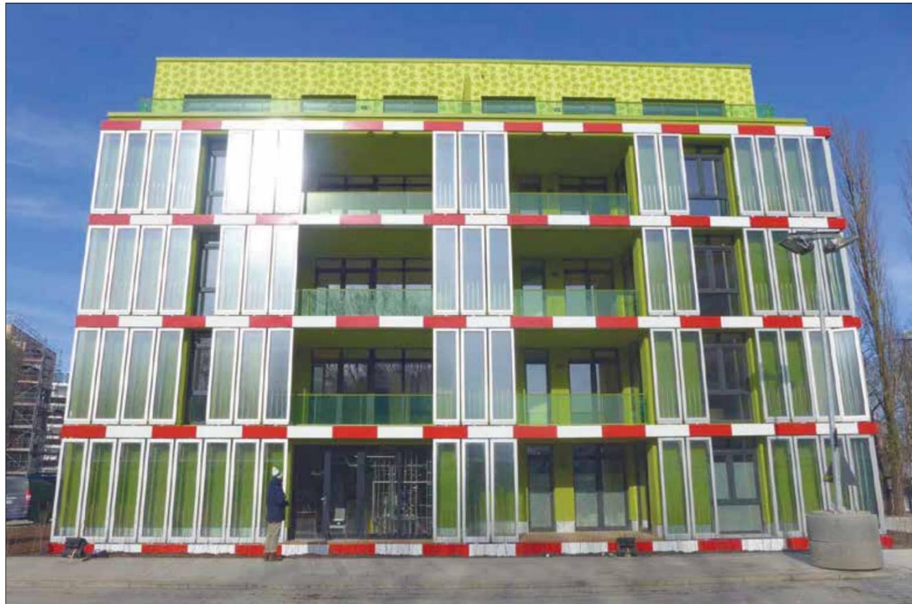
The vertical glass louvres of the four-storey Hamburg apartment block have been filled with water and nutrients through which microalgae circulate, converting daylight and CO<sub>2</sub> to biomass and solar thermal heat through photosynthesis © Colt International, Arup Deutschland and SSC Strategic Science Consult
