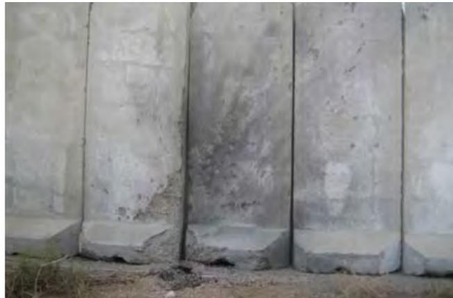
Damage to a T-Wall barrier caused by a 120mm Rocket fired at Basra International Airport by Iraqi insurgents © Major Sean Matten
