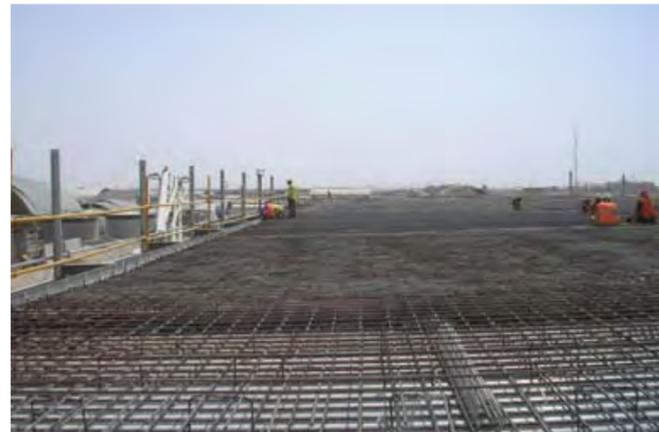
The roof of a permanent reinforced concrete Dining Facility (DFAC) being constructed on the COB by KBR (UK) © MOD
