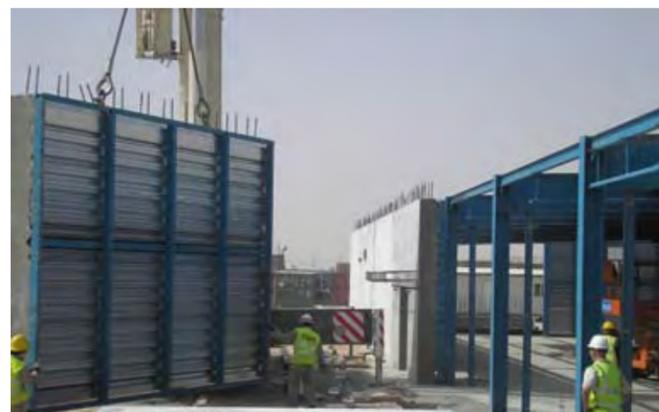
Prefabricated wall sections of a permanent dining facility being moved into place. Virtually all fabrication was conducted within Basra International Airport © MOD
