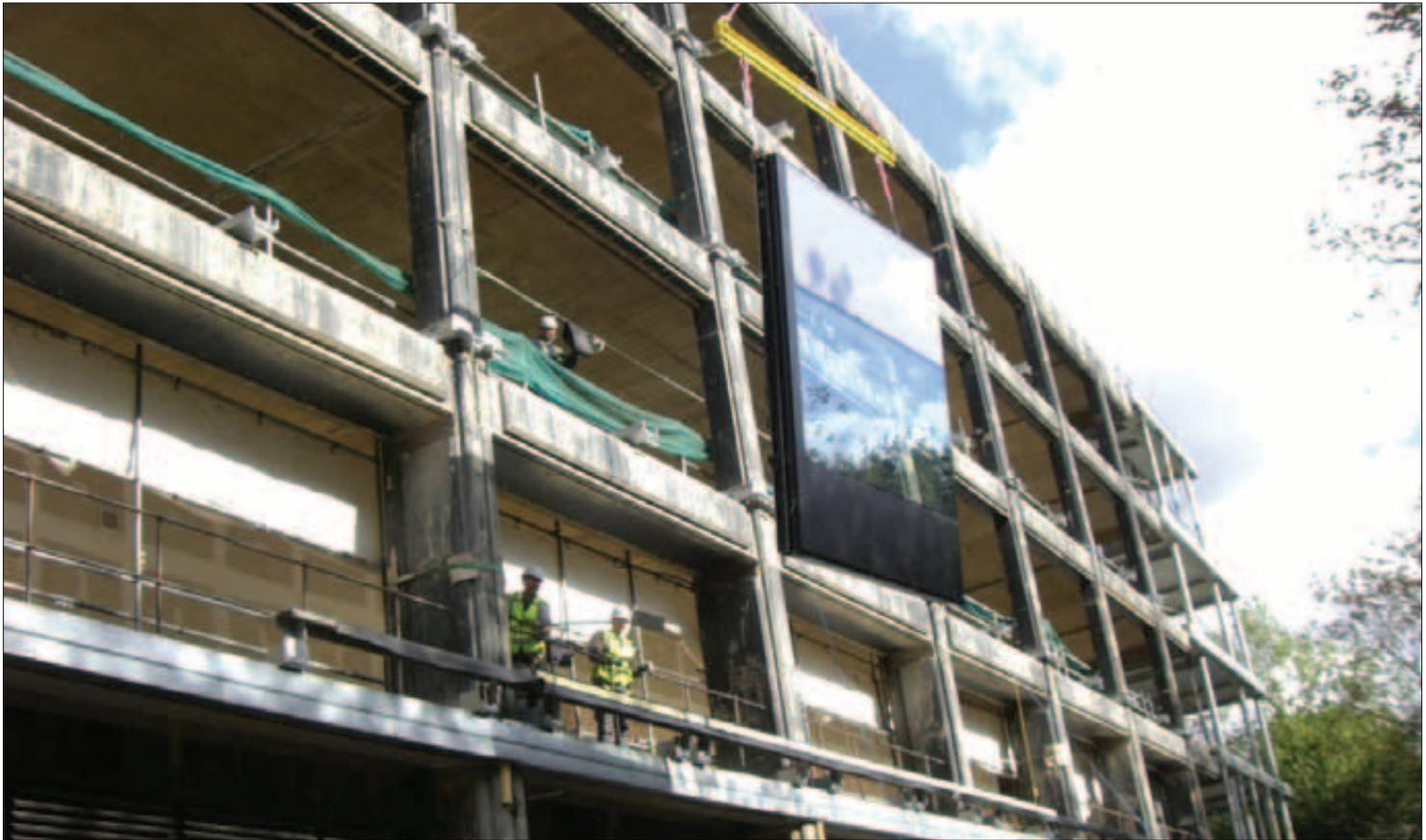
The first panel goes onto the renovated Angel Building in Islington, north London. The unitised panels installed were prefabricated complete with glazing, insulation and finishes. Fixing brackets were installed to the slab perimeter in preparation for receiving the unitised panels © Allford Hall Monaghan Morris
