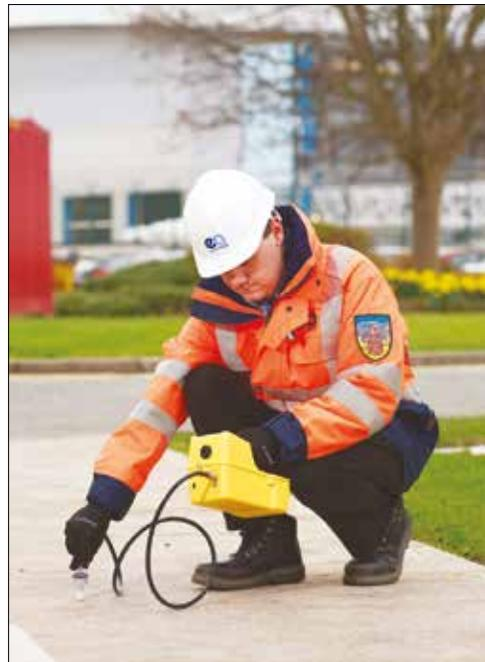
A CableSniffer is inserted into test holes looking for gases emitted from the burnt cable insulation of a low-voltage cable
