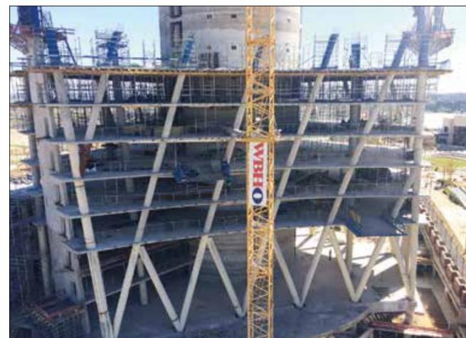
The chosen arrangement of columns under construction, with five across the width of the facade and repetition every five floors. Each column is spiral in shape, but made up of storey-height straight sections with changes of angle at each floor. The counter-sloping columns are purely architectural – to create a V pattern at the lobby level – and carry no loads © Arup
