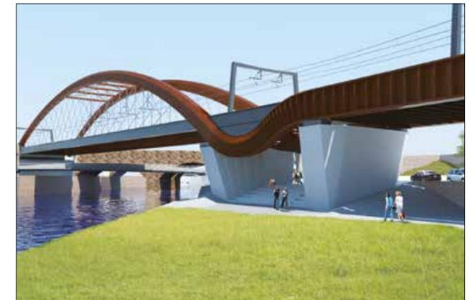
Visualisation of the proposed network arch bridge over the River Irwell which forms part of Network Rail's planned Ordsall Chord, a short section of new railway in central Manchester. The bridge will be built in weathering steel to reduce long-term maintenance requirements. The varied thickness of the steel plates used means that its area is roughly constant and the asymmetry in its behaviour is reduced
