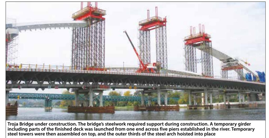
Troja Bridge under construction. The bridge's steelwork required support during construction. A temporary girder including parts of the finished deck was launched from one end across five piers established in the river. Temporary steel towers were then assembled on top, and the outer thirds of the steel arch hoisted into place
