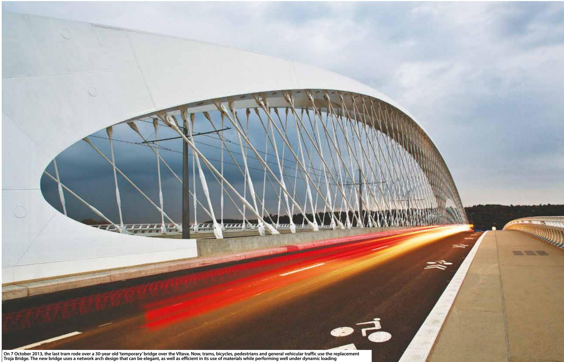
On 7 October 2013, the last tram rode over a 30-year old 'temporary' bridge over the Vltava. Now, trams, bicycles, pedestrians and general vehicular traffic use the replacement Troja Bridge. The new bridge uses a network arch design that can be elegant, as well as efficient in its use of materials while performing well under dynamic loading
