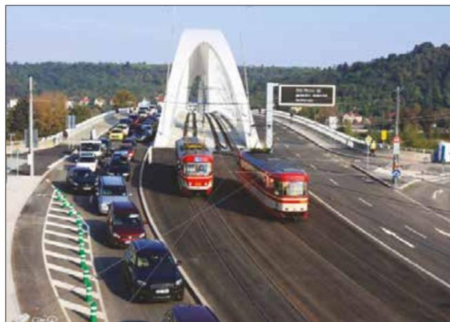
The full 35m-width of the Troja bridge supports four lanes of traffic plus cycleways and footpaths, with the twin tramlines at the centre to minimise eccentric loading. The arch splits towards the ends into four legs to allow the trams to pass through
