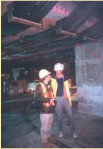
Figure 7 Antidrag system (ADS): upper level of tunnel shield (indicated) showing anti-drag ropes just behind roof exit slots
