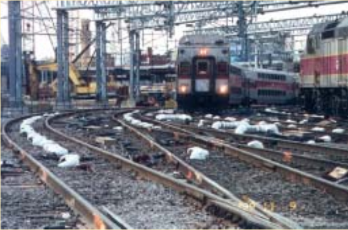
Figure 5 Ground freezing under railway
