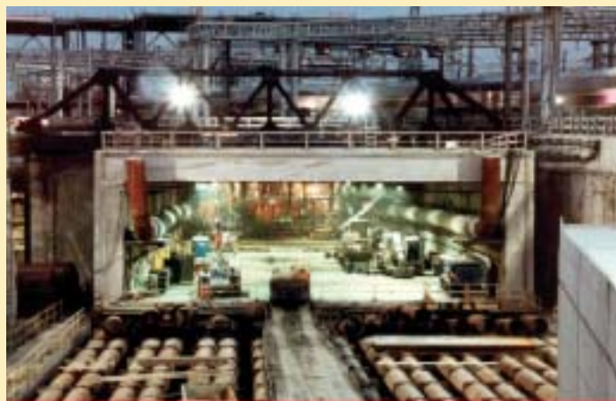
Figure 2 I-90 Eastbound jacked tunnel
