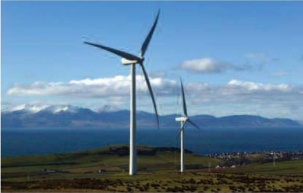
Airtricity's first Scottish wind farm which consists of 12 V80 2MW turbines © EMPICS
