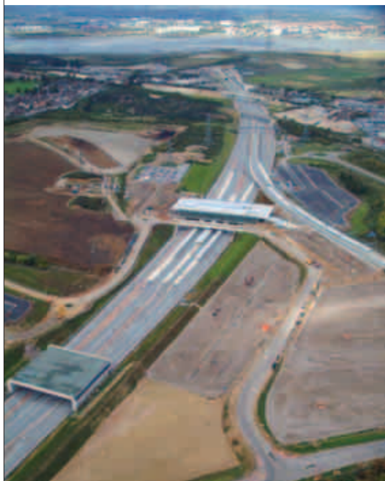
Ebbsfleet International Station under construction © Hawk Editions/LCR
