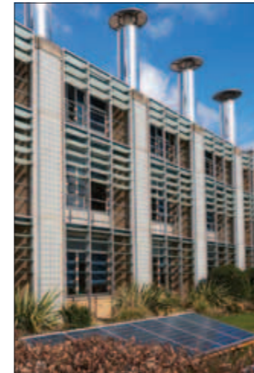
The BRE Environmental Office, completed in 1996, was one of the original smart buildings. It includes thermal mass cooling and solar-driven extract chimneys © Doug King
