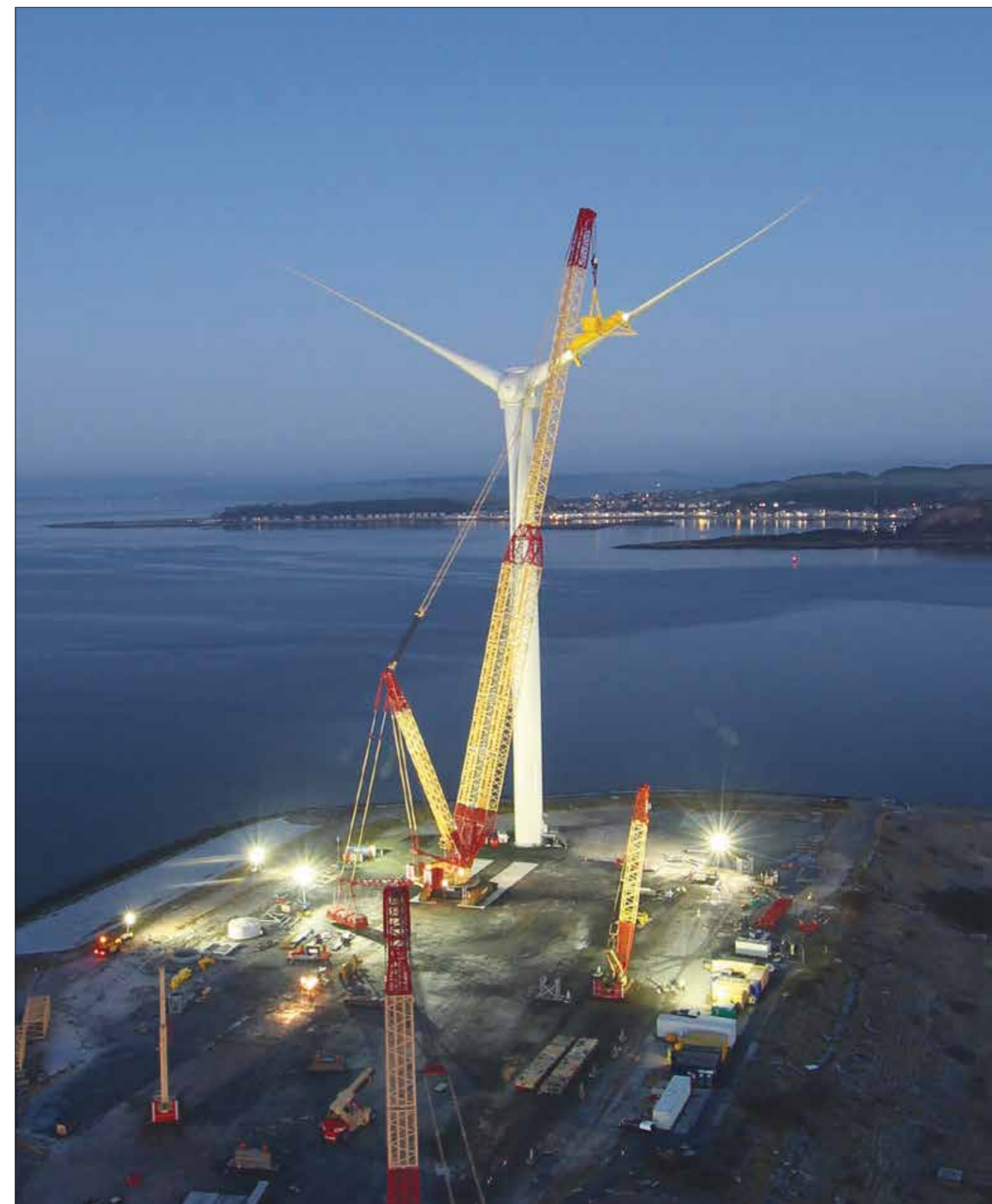
Onshore verification testing of a digital hydraulically driven offshore wind turbine at the Hunterston Test Centre by the Firth of Clyde. The rotor diameter is 167m © MHI
