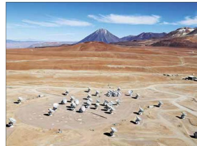
ALMA from the air. The array consists of 66 antennas situated on the Chajnantor Plateau at an altitude of 5,000 m in the Chilean Andes. The large antennas have a diameter of 12 m, while 12 smaller antennas have a diameter of 7 m © Clem and Adri Bacri-Normier (wingsforscience.com)/ESO
