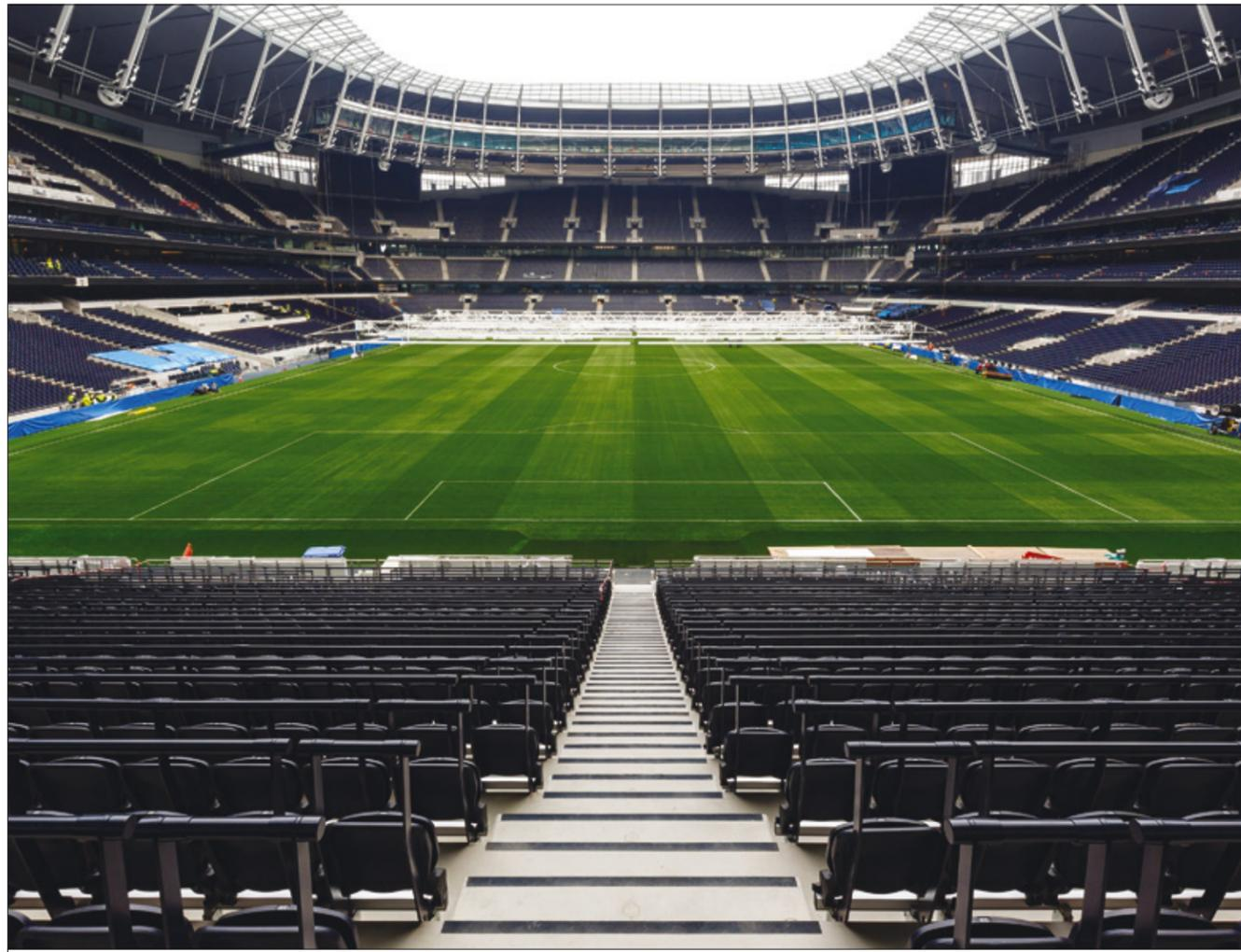
The football pitch at the new Tottenham Hotspur Stadium hides an artificial NFL field underneath. The pitch slides over in three metal trays, each weighing over 3,000 tonnes, which are stored beneath the stands when not in use © Tottenham Hotspur / SCX Special Projects
