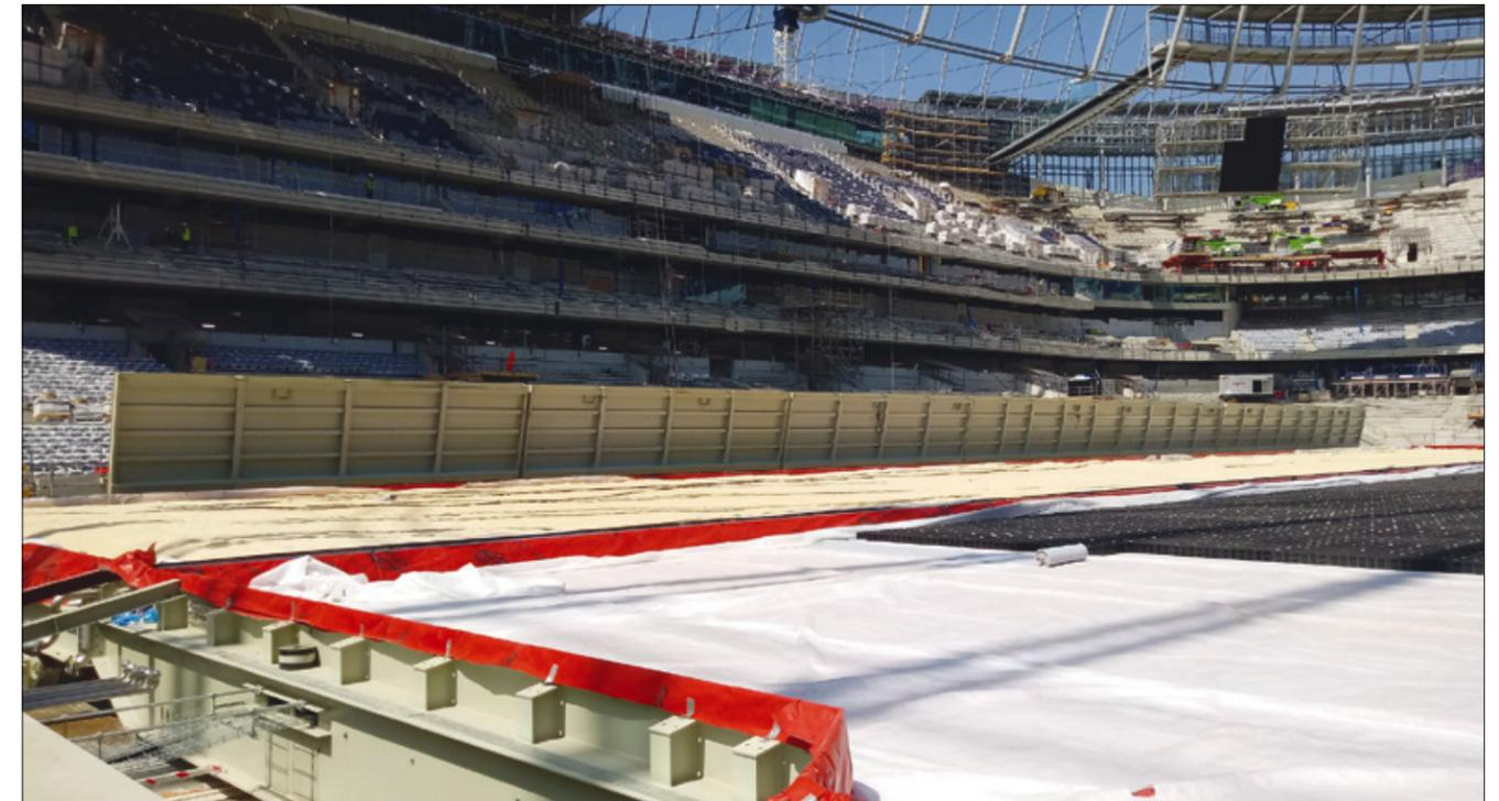
When the NFL pitch is in use, the touchline structure lowers to ground level and the flaps sit flush on the side of the artificial pitch. When the pitch sections are ready to be rolled in, the flaps can be raised into a vertical position at the touch of a button © Tottenham Hotspur / SCX Special Projects
