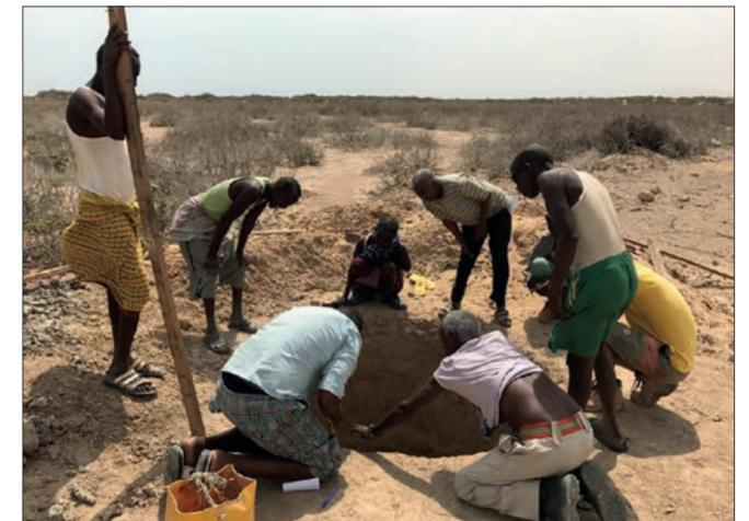
Beach wells, 200 metres from the beach, use sand to clean and filter water before it is pumped to the grow-house © Seawater Greenhouse Ltd
