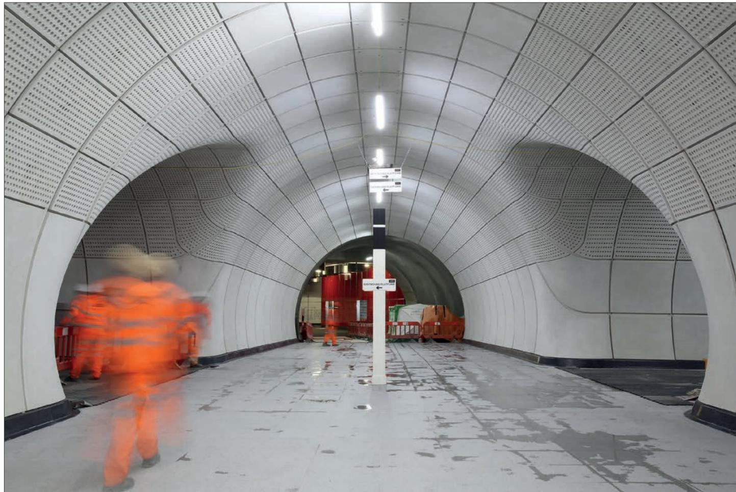
The fitting out of the Elizabeth Line stations on the London Underground included the creation and installation of glass fibre reinforced concrete cladding panels. These were used to negotiate and accommodate complex shapes as well as to ensure structural strength © Crossrail
