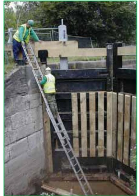
**Figure 1 Refurbishment work on the Manchester Rochdale lock**
