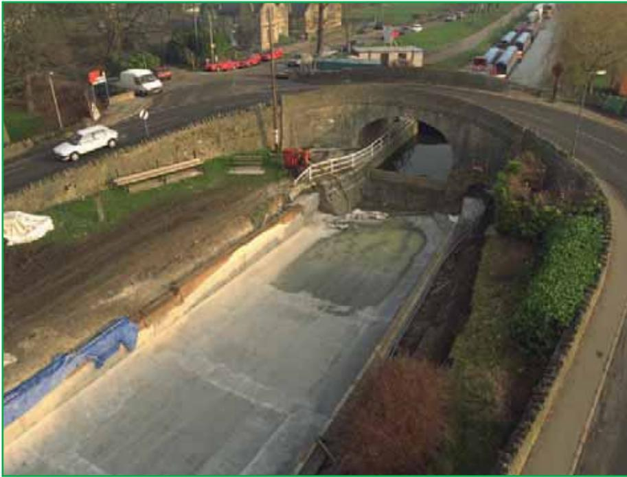
**Figure 2 Relining a stretch of the Kennet & Avon Canal near Bath**
