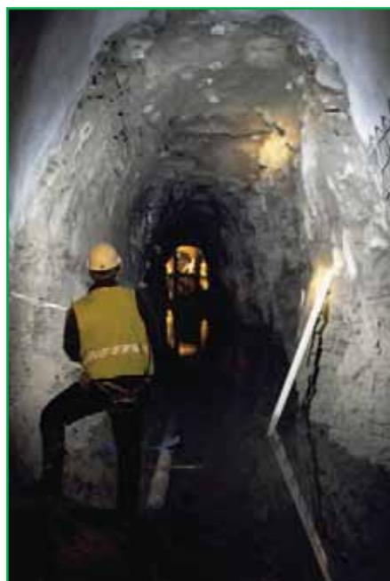
**Figure 7** Relining of the Standedge Tunnel
