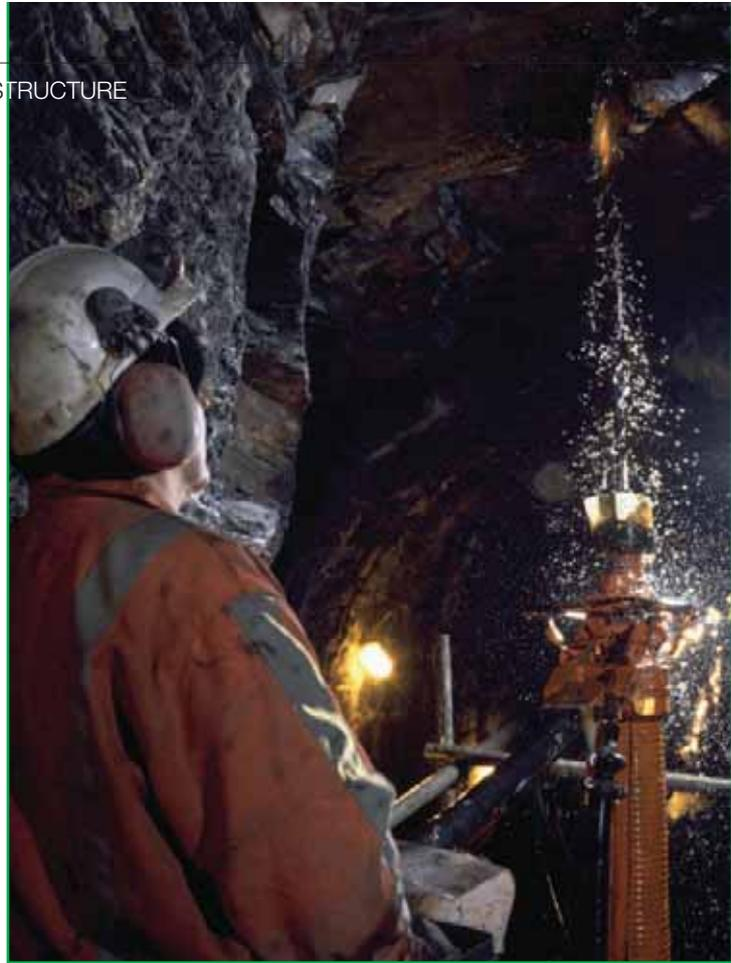
**Figure 8** Rock bolting of Standedge tunnel
