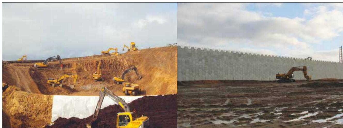
Before construction could begin on the Shetland Gas Plant, a substantial amount of earth was moved. The soil and peat that was excavated was used to extend the terracing of the bedrock and two large peat stores were designed and created to accommodate the material so that the peat can be recycled to restore the site to its predevelopment condition at the end of the plant's life © Total
