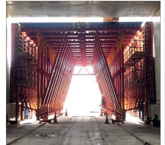
Travelling formwork for constructing the 11,000 t 155 m-long concrete portal before it was jacked into place © eb7 Immersive
