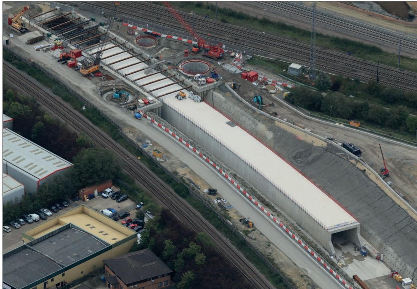
The 155 m-long concrete portal almost complete, before the start of jacking
