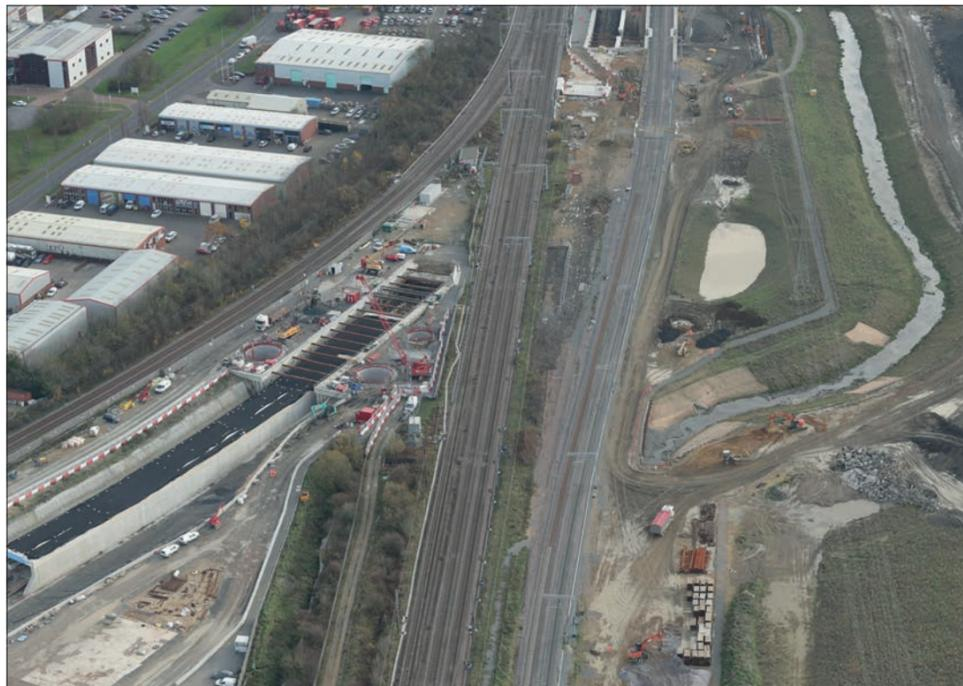
The site at Werrington last November showing the East Coast Main Line running southwards towards Peterborough and London King's Cross, the Great Northern Great Eastern freight lines joining at a flat crossing from the left, and the (already diverted) Stamford lines running parallel to the ECML to the right. The curved concrete portal is under construction alongside the freight lines, with the reception area and ramp just to the right of the ECML beyond
