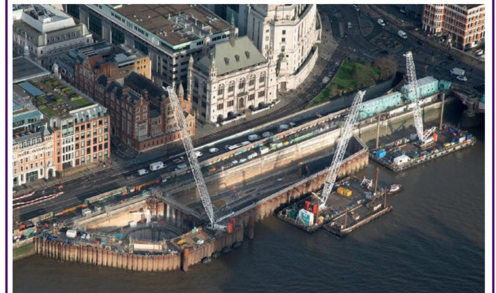
Blackfriars north foreshore. A 100-metre, 3,500-tonne interconnecting culvert will be the largest structure to pass along the Thames later this year. It will be lifted into the central section above and then connected to the CSO drop shaft – below the crane on the left of the picture © Tideway
