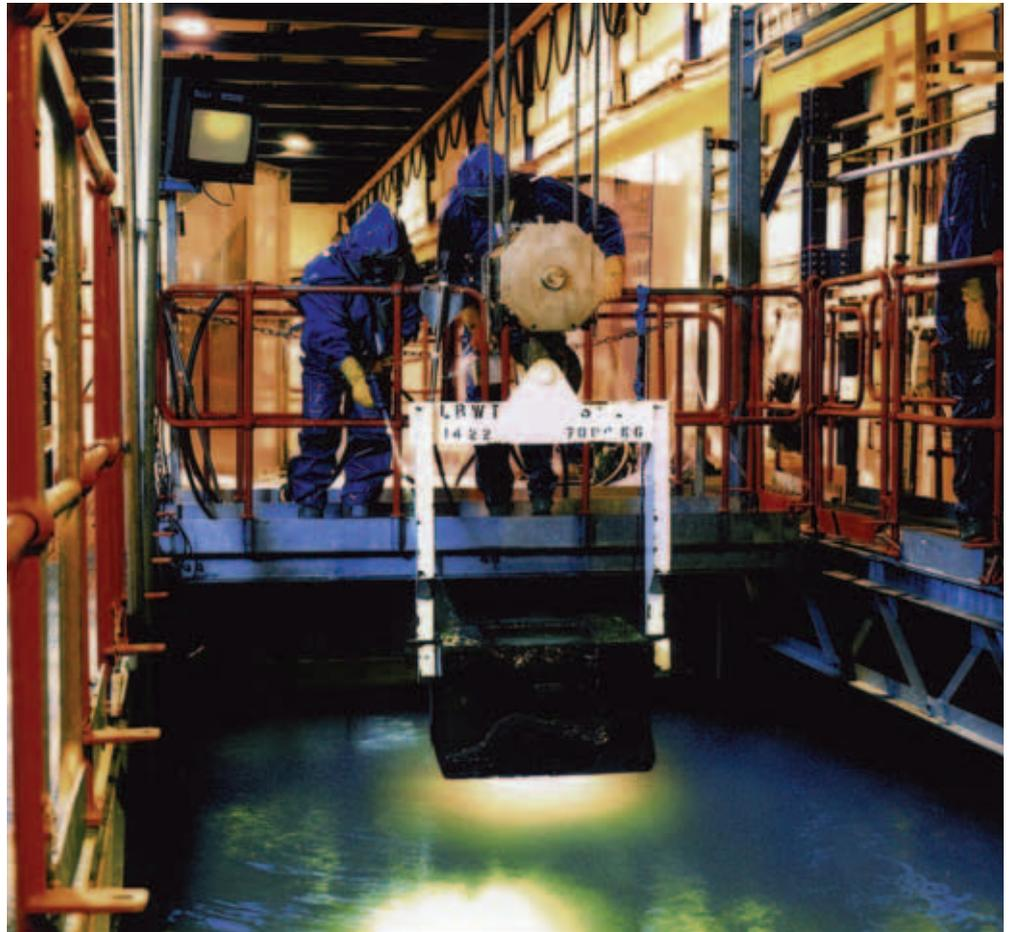
Removal of a redundant uranium storage flask from a storage pond at Sellafield © NDA
