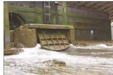
One of more than 50 combined sewer overflows which, on an average of once a week, discharge untreated sewage and storm water into the River Thames in London, a total of 40 million tonnes a year © Thames Water
