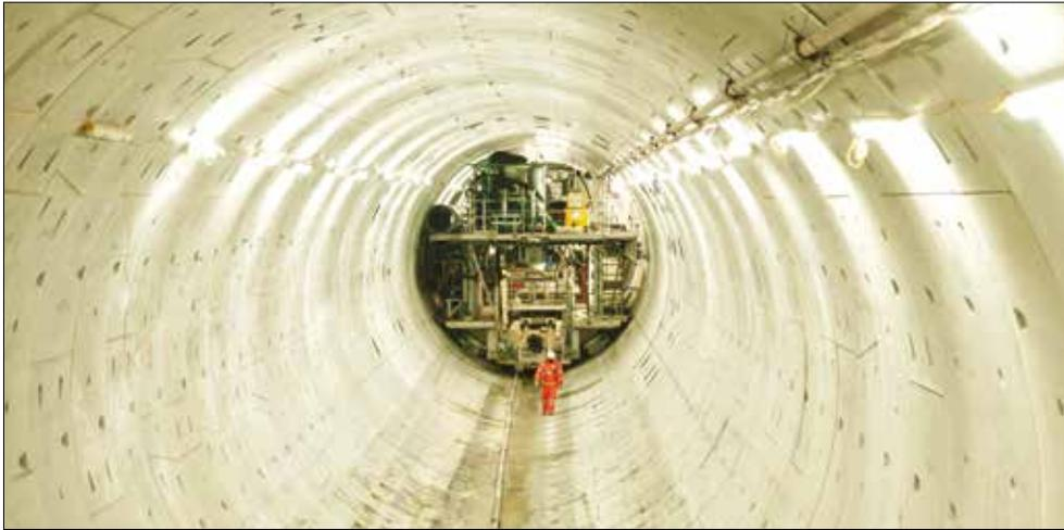
The primary segmental tunnel lining at 7.8m internal diameter is erected by the TBM itself. Here the back of the TBM can be seen after the initial short tunnel drive and during the extension of the machine to its full 120m length prior to commencement of the remainder of the 6.9km tunnel. © Thames Water
