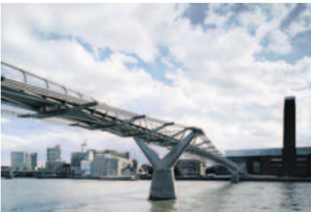
under approximately 1.3 Hz, with enough pedestrians on the bridge in relation to its mass and damping.
