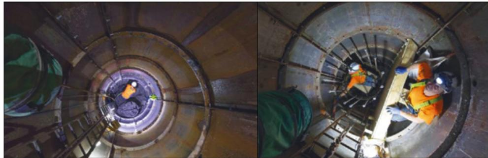
A miner hand excavates one of the 61 steel-lined caissons (left), while another places a reinforcing bar for a new column within the tight space of a hand-dug caisson (right) © McGee
