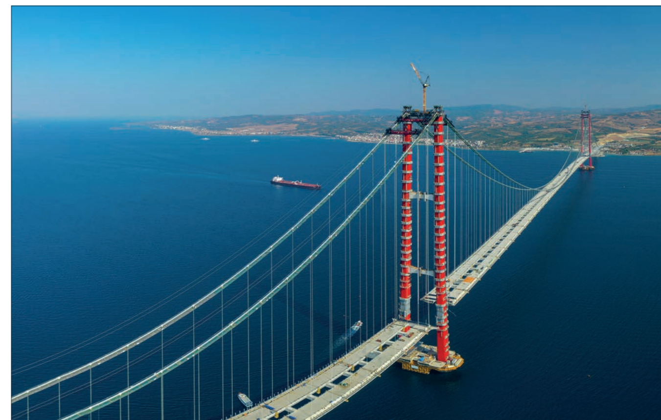
The 1915Çanakkale Bridge during construction of the central deck section © Shutterstock
