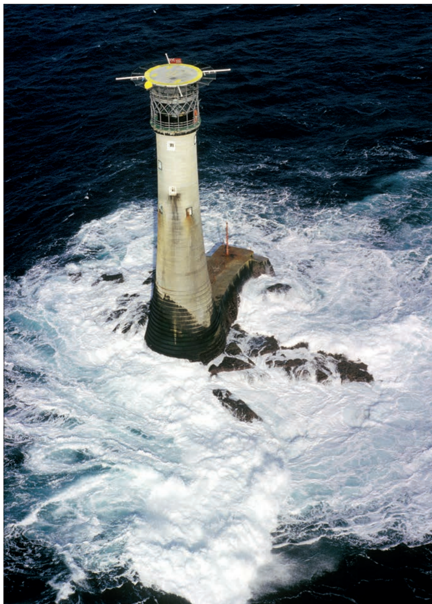
Wolf Rock lighthouse, a 19 th -century offshore, rock-mounted structure off Land's End, was the focus of a project looking at the future integrity of such at-risk structures © Alamy
