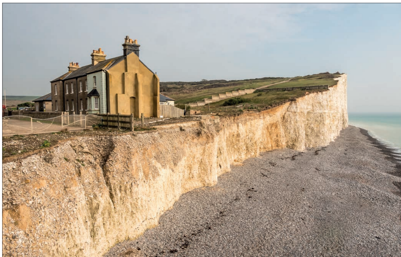
Erosion at Birling Gap, in Sussex. Several houses have been demolished, instead of being allowed to collapse over the cliff edge © pxl.store / Shutterstock
