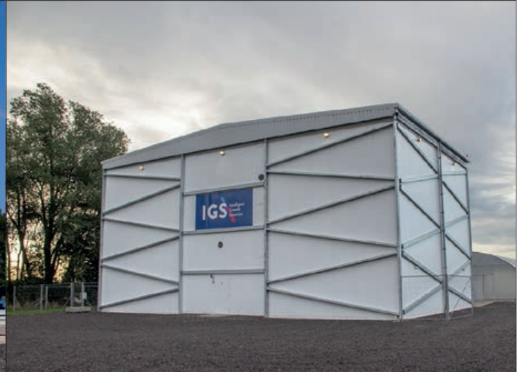
The Dundee farm is housed in a purpose-built superstructure that has insulated cladding to protect crops from the external environment. The structure has space for four growth towers © Intelligent Growth Solutions
