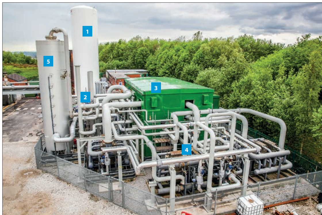
1. Liquid air storage 2. Cryo pumps 3. Power turbine and generator (5 MW) 4. Heat exchanger containers 5. High grade cold stores © Highview Power
