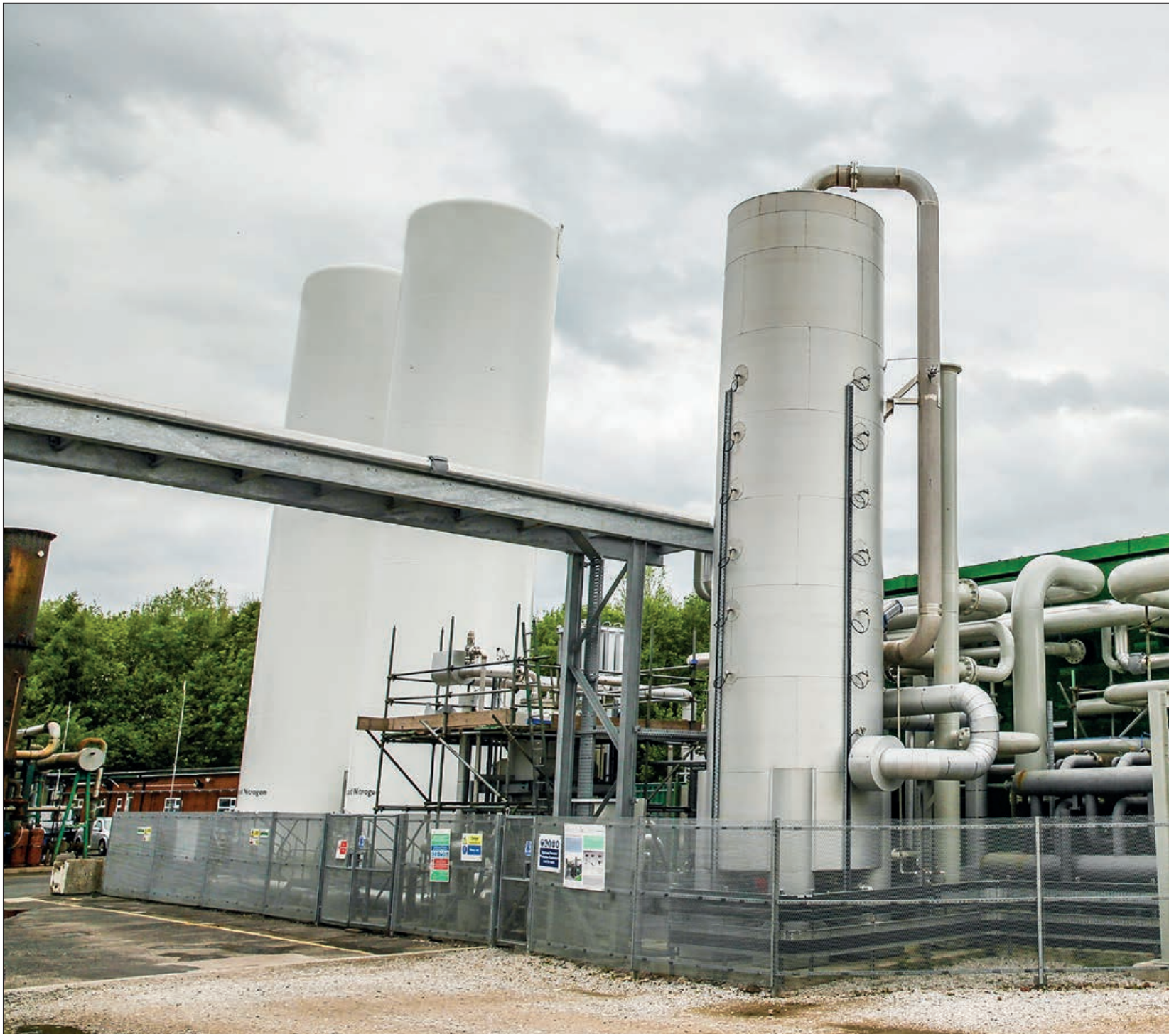
The 15 MWh cryogenic energy storage demonstration plant at Bury commissioned in 2018 © Highview Power
